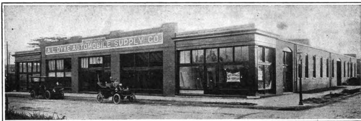
A TYPICAL AUTOMOBILE HEADQUARTERS IN THE CITY OF SAINT LOUIS.
